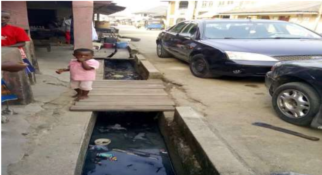
Fig,2.3: Municipal drainage in Emeyal 2 community
